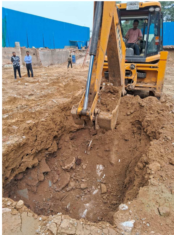
PHOTOGRAPHS SHOWING VIEW OF THE SITE AND BOREHOLE UNDER PROGRESS
