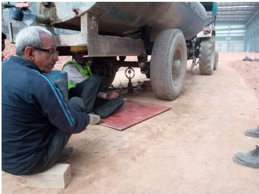
PHOTOGRAPHS SHOWING PLATE LOAD TEST UNDERPROGRESS
